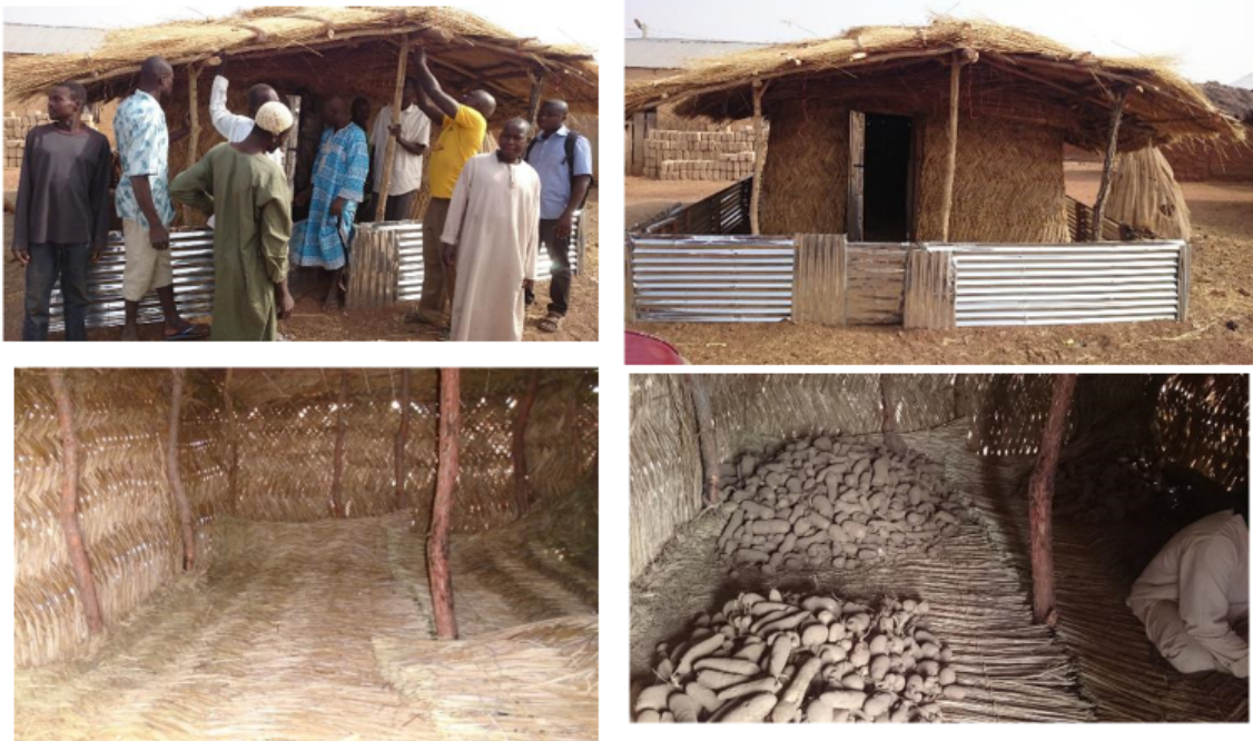
Fig.7. Improved storage structure fenced with roofing sheets to eliminate rodents. The thatch roof also prevents rain water from entering the structure
